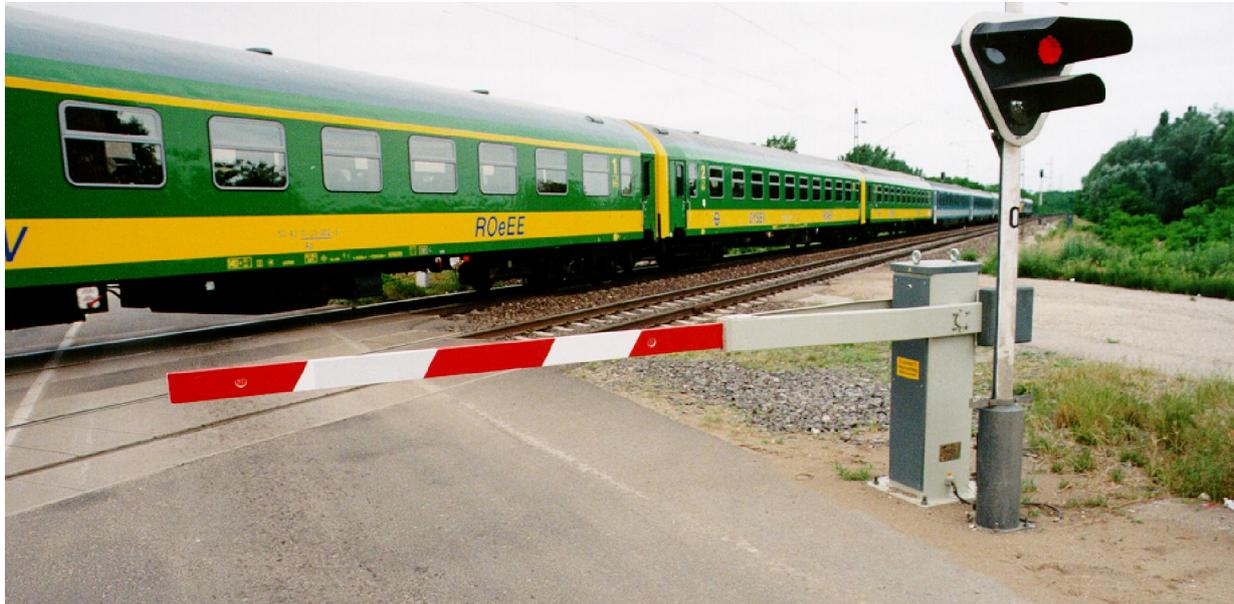
MA-HSH-03 type hydraulic crossing barrier drive is an electrically controlled and pneumo-hydraulically driven construction. The basic tasks of the barrier drive are the physical locking of road traffic in the road-railway level crossings by controlled way, the illumination of the barrier boom by flashing light and the check-back of the barrier boom position.
